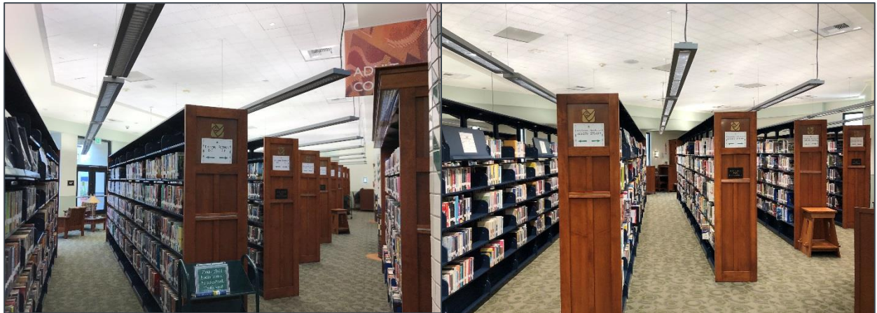
Figure 3: Before (left) and After (right) Book Stack Lighting Retrofit at Serra Mesa-Kearny Mesa Source: CSE and City
